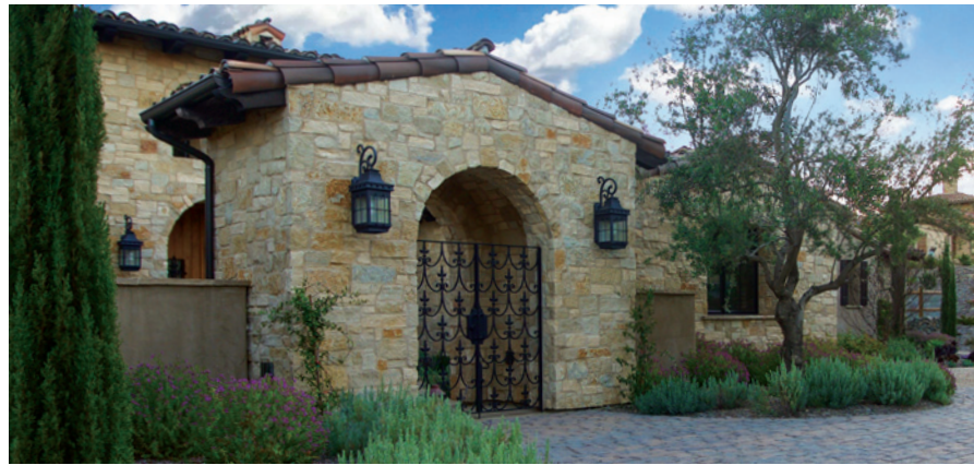
TUSCAN BLEND RUBBLE INSTALLED WITH A STANDARD RAKED MORTAR JOINT
