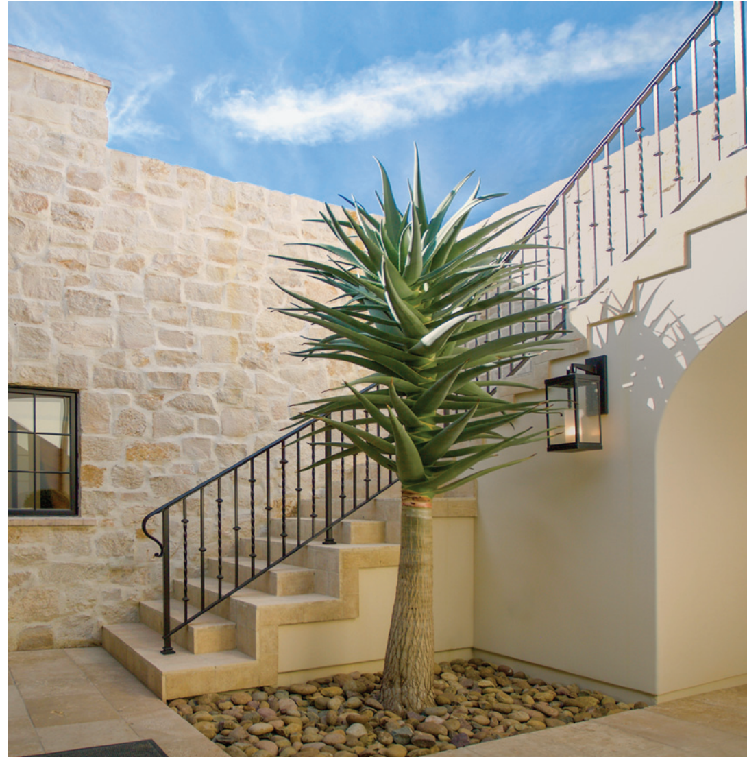
ABOVE: HONEY BUFF RUBBLE INSTALLED WITH A MORTAR WASH TECHNIQUE RIGHT: TUSCAN BLEND RUBBLE WITH NO-RAKE MORTAR JOINT
