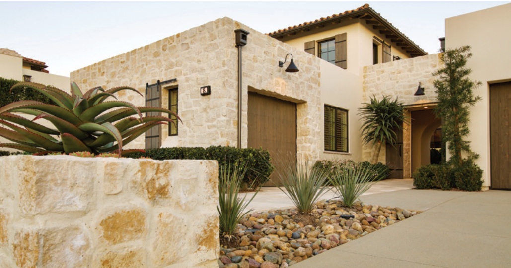
ABOVE: HONEY BUFF RUBBLE INSTALLED WITH A MORTAR WASH TECHNIQUE RIGHT: TUSCAN BLEND RUBBLE WITH NO-RAKE MORTAR JOINT
