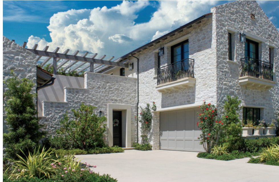
TUNDRA CREAM RUBBLE INSTALLED WITH A MORTAR WASH TECHNIQUE
