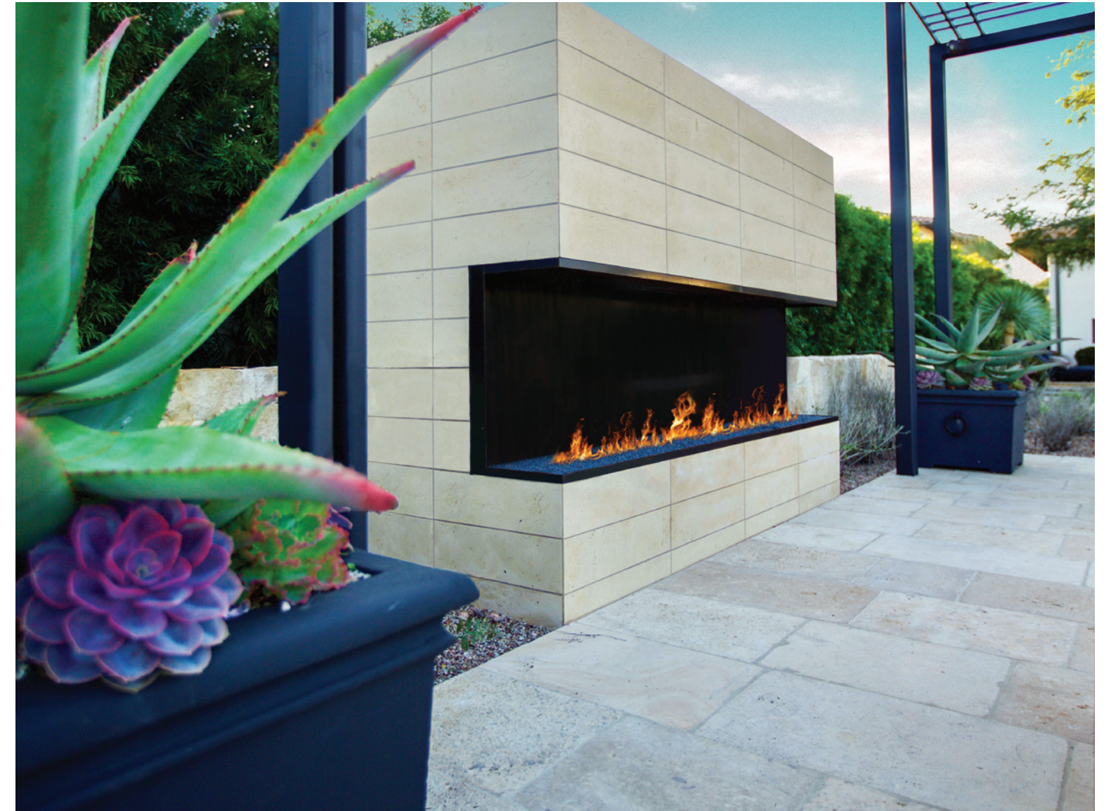
NADIA NEO PLANKS INSTALLED WITH A FLUSH MORTAR JOINT
