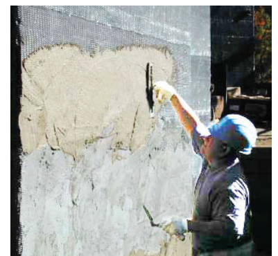
FIG.1A-ATTACHING LATH, FIG.1B-APPLYING SCRATCH COAT OF MORTAR
